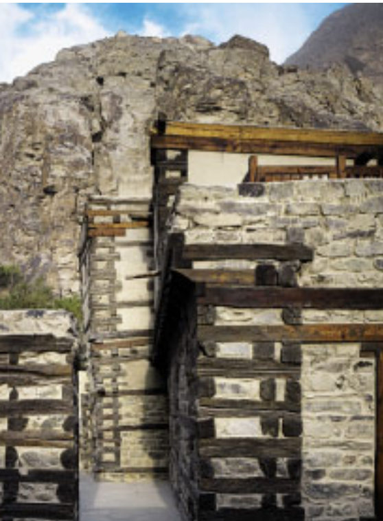
Altit Fort is typical of building construction in the Gilgit-Baltistan area, with reinforcing cribbage structures at the corners and horizontal cators stabilizing the walls.
